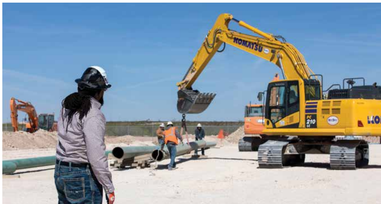
Brazos Midstream pipeline construction stretching Reagan, Glasscock, Midland, Martin, Howard, Andrews, and Ector counties in the Midland Basin. Pipeline construction is an imperative in the Permian Basin as output is rapidly reaching capacity.
